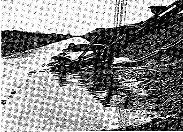
LAND RECLAMATION. — EXCAVATOR AT WORK.
